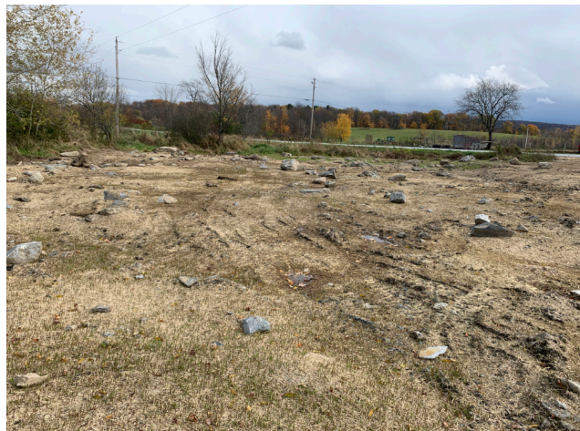
Post restoration-fill removed, rough finish incorporating boulders
