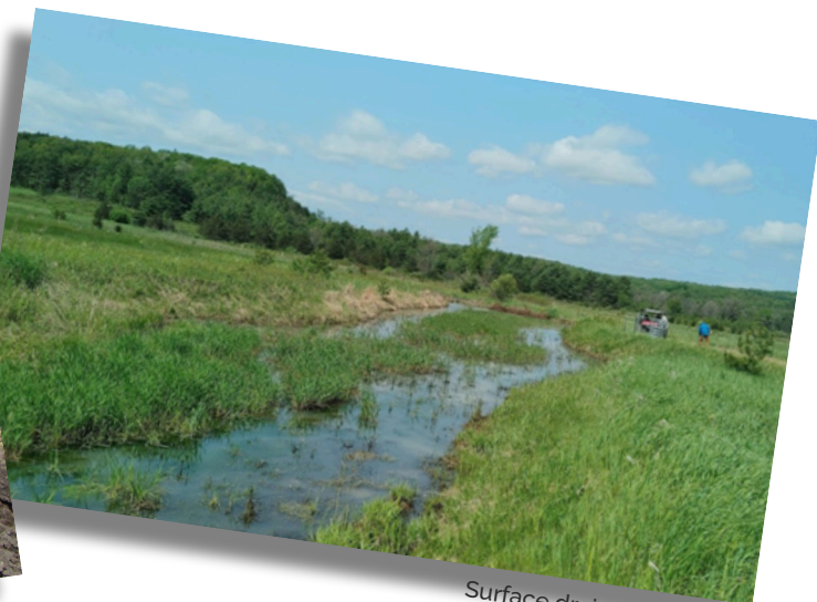
Surface drainage reroute, Shayne Jaquith, TNC
