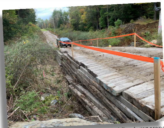
Layered wetland matting providing temporary wetland crossing
