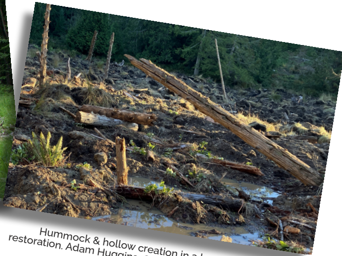
Hummocks & hollows constructed in a small sloped forested wetland restoration
